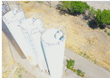
Pirelli Tanks, Colusa 1 Radio
