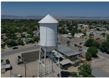
Williams Water Tower Railing - 4 Radios
