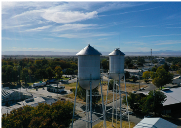
Colusa Reclamation District Tower - 2 Radios
